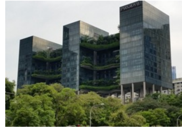
"Green" Building in Singapore, Courtesy Brian Meacham.
