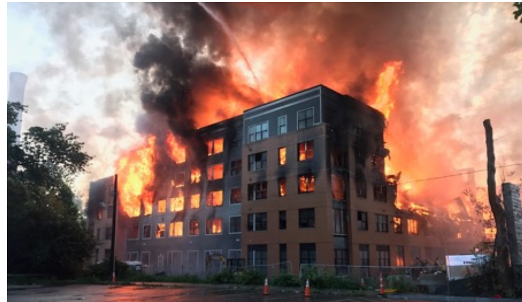
Fire in Timber Frame Apartment Building Under Construction (Source: Captain John Bonadio, Waltham Fire Department, as published at https://www.enr.com/articles/42484-what-local-officials-want-to-do-about-wood-frame-building-fires-in-massachusetts ), Courtesy of Waltham, Massachusetts Fire Department)
